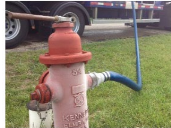
Figure 1. A typical set up for inserting ice into a water main pipeline using a hydrant and two-and-a-half-inch fire hose.
