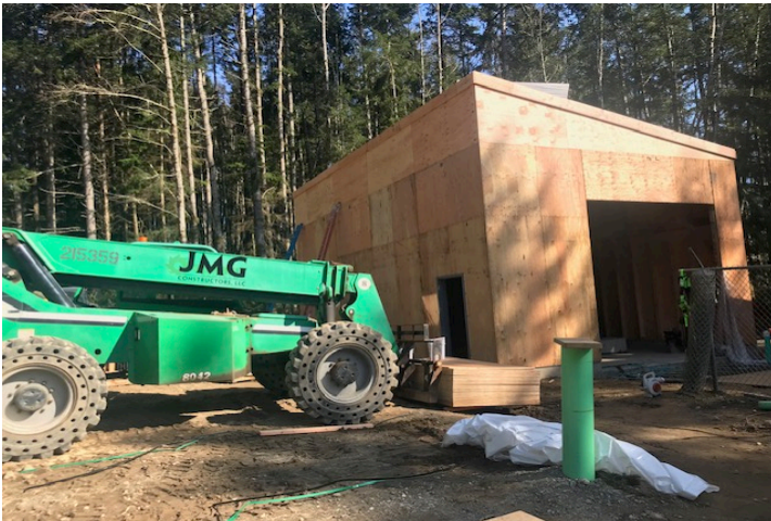
The building is going up rapidly and will have siding installed this week.
