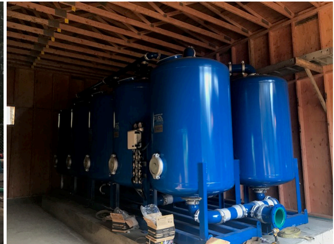
The filters are under cover.
