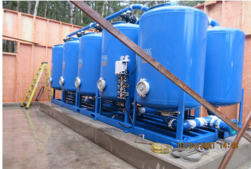
The filters placed on their concrete pad.
