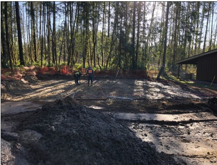
Site is cleared. Building foundation is being laid out.
