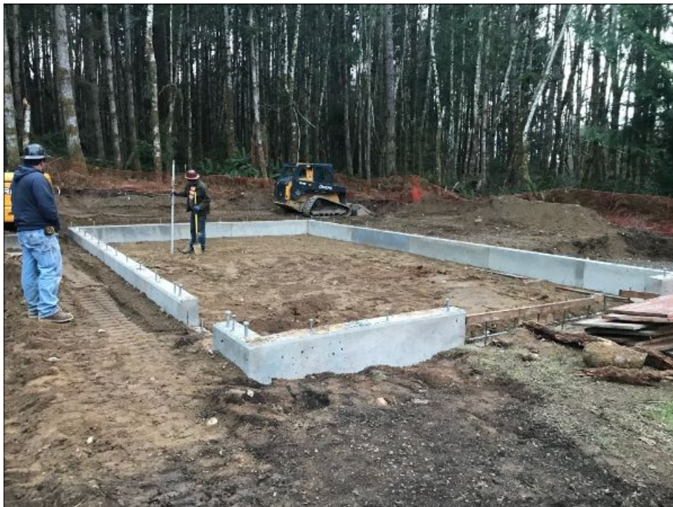
Filtration Building, January 22, 2021
