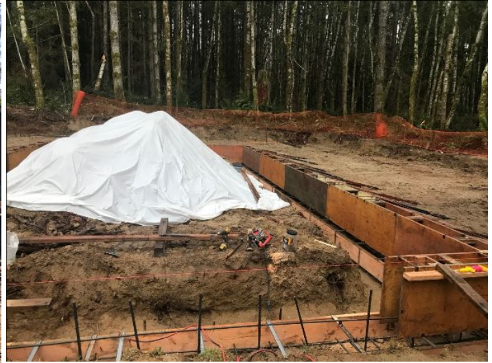
January 19 Filtration building forms are ready for concrete.
